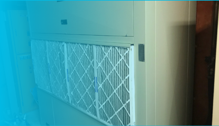
New cooling tower and WC package unit
